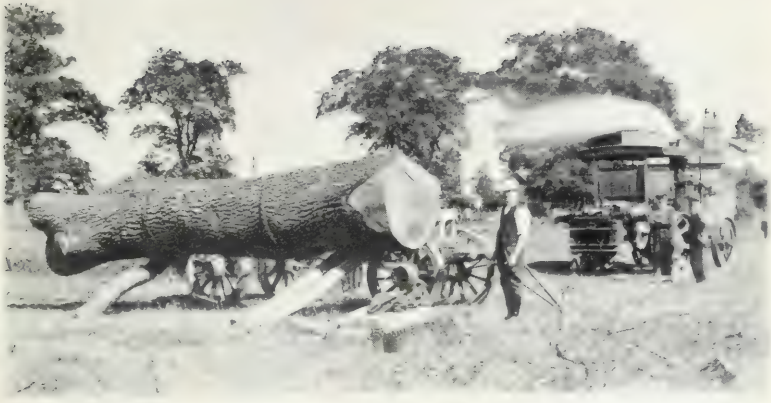
FIG. 43. STEAM WAGGON LOADING LOG BY CROSSHAUL.
